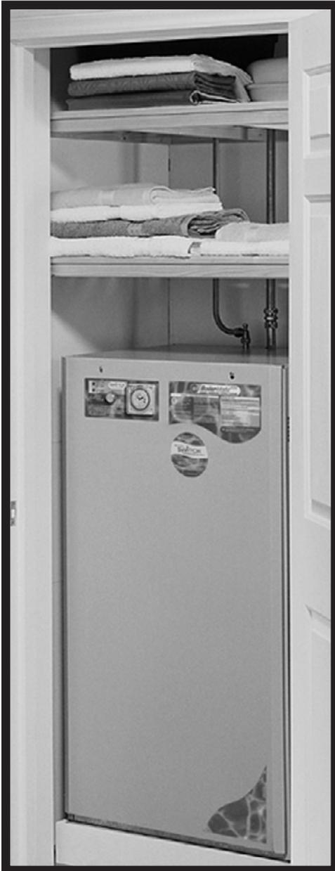
Your BoilerMate 2000 is a highly advanced Thermal Storage System which incorporates the latest in microprocessor technology to monitor your system automatically and ensure it operates at maximum efficiency. This includes periodically 'spinning' the heating pump to prevent seizing during prolonged unused heating periods.
